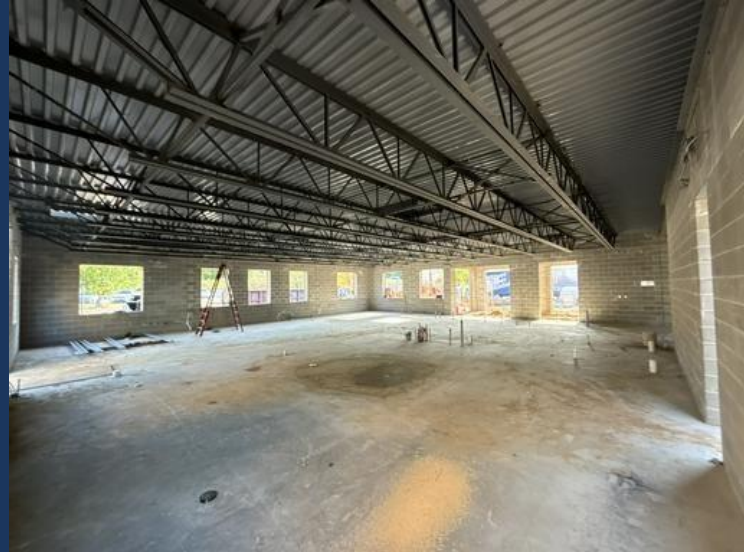
View from inside new addition
